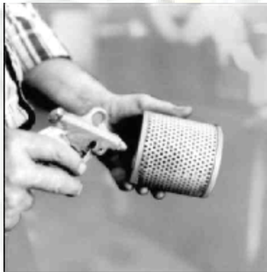
Cleaning the air filter
